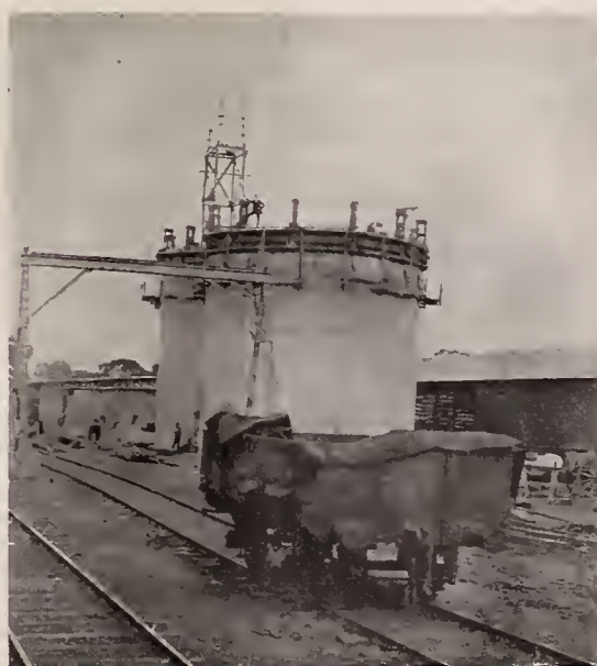
100,000 BUSHEL ELEVATOR UNDER CONSTRUCTION AT URANQUINTY
